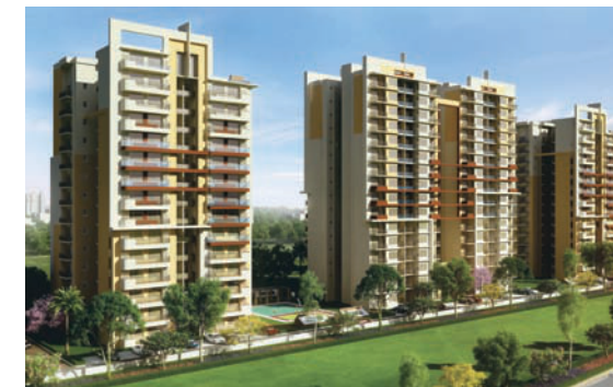
GREEN LOTUS AVENUE - CHANDIGARH AMBALA HIGHWAY -
